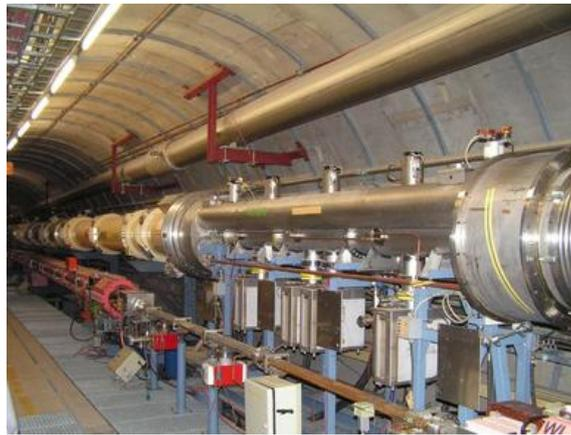
**Figure 29.** Kicker bypass in the HERA tunnel (West left 200 m). The bypass will be installed in the middle of the experiment connecting the two dipole strings of ALPS-IIc and pass the magnet current and the cryogenics around the optical setup.
