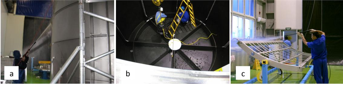
**Figure 8.** (a) Pressure cleaning of the outside of the SSV. (b) Cleaning the interior of the SSV. (c) Pressure cleaning of a PMT ladder..
