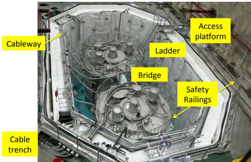
**Figure 18.** A near hall nearing completion. The access platform and ladder provided access to the top of the detector where final gas and electrical connections were made. Railings around the AD and pool protect workers from the 7-10m drop to the pool floor. The cableway running around the pool and the cable trenches outside the pool are also shown.
