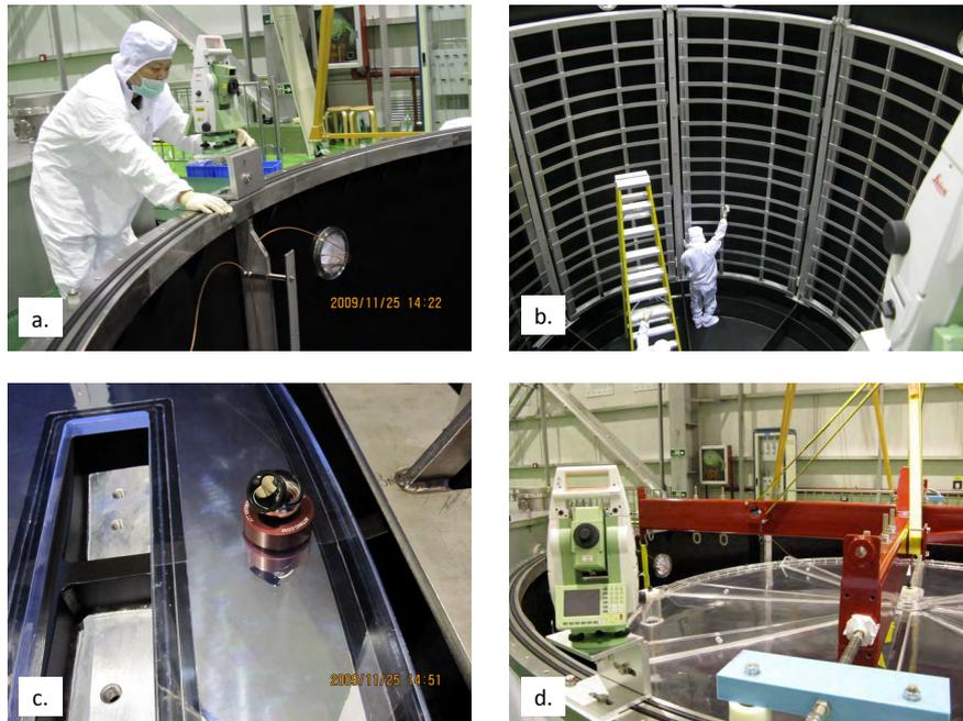
**Figure 12.** (a) Setting up Total Survey Station on SSV flange. (b) Measuring radius of PMT ladders. (c) Survey of height of lower reflector. (d) Adjusting the position of the OAV to align the central port with the SSV.
