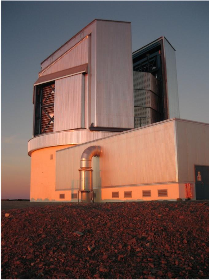
**Fig. 14.** VISTA enclosure seen from the southwest at sunset, with the auxiliary building in the foreground. Here the wind-screen is fully raised, and an open ventilation door is seen on the left.
