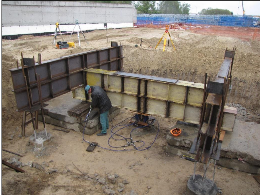
Figure 1. Boryspil Pile #3 test view
