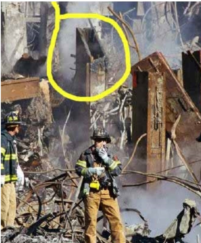
Figure 2: Photograph taken after collapse of the WTC towers. Enclosed in the yellow circle is a column with a straight cut. Source: public domain.
