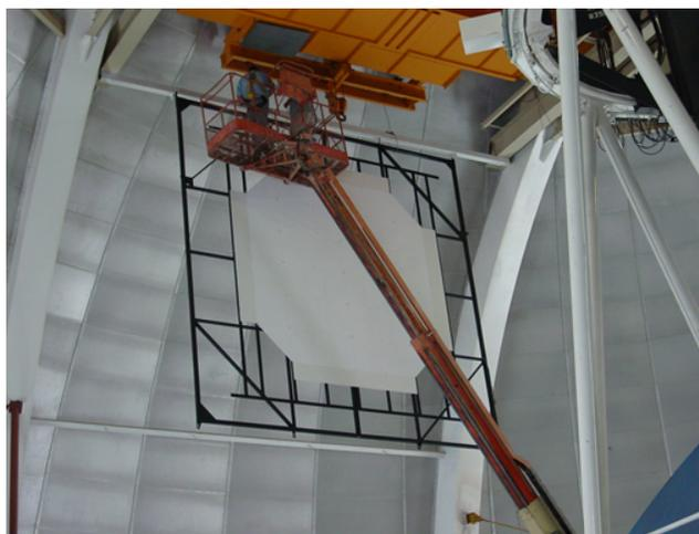
**Figure 8.4:** Installing the existing reflection screen used for daytime flat fielding. The screen is being mounted to the inside of the dome, between the arch girders and just below the attachment point for the dome crane rails. Note the use of a long-reach boomlift. For safety reasons, the telescope drives must be locked out and tagged out during the entire operation.
