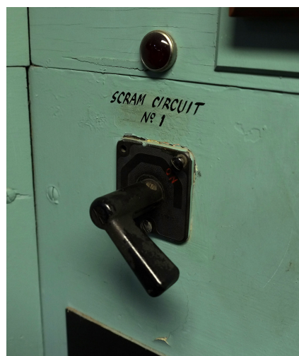
Figure 1.1: SCRAM button in the control room of the X-10 Graphite Reactor at Oak Ridge National Laboratory.
