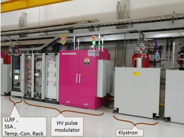
Figure 3 : Picture of a RF station
