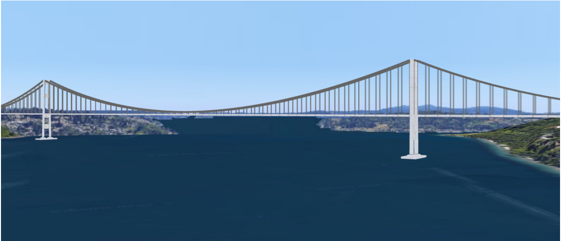
FIGURE 1. A typical suspension bridge with two towers and three spans.
