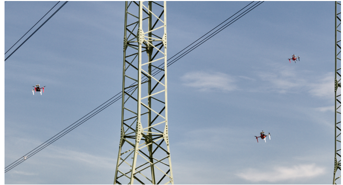
Figure 1. Our MRS research platforms [2] capable of performing visual inspection on a power transmission line. Source: Neugebauer, CTU in Prague.
