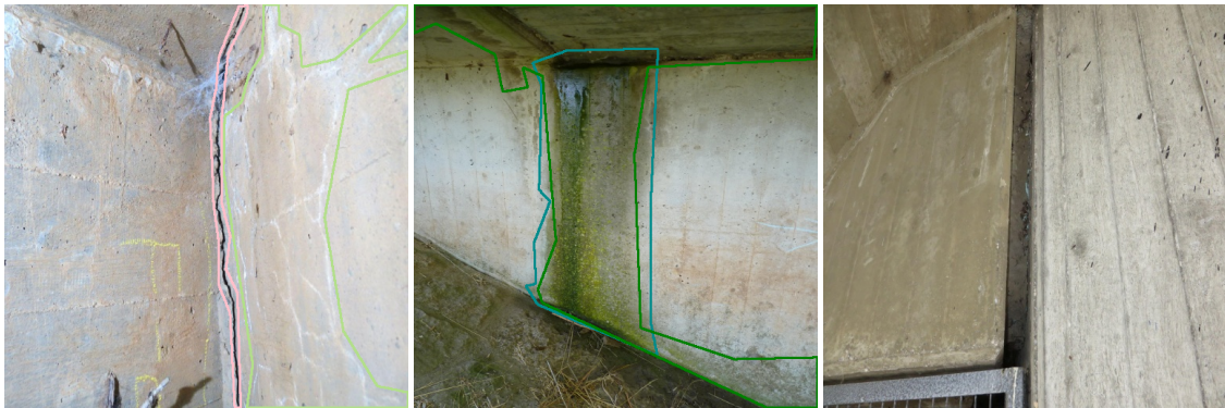
(b) Crack vs. Alligator Crack , Weathering vs. Wet spot , Restformwork covered with concrete slurry (no ground-truth annotation for better visibility).
