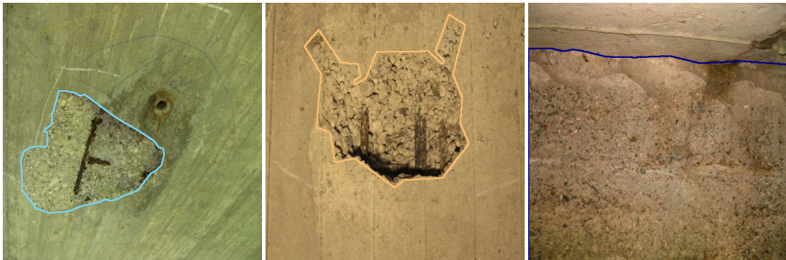
(c) Spalling , Rockpocket , Washouts/Concrete corrosion .
