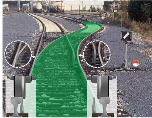
Fig. 3. Close-up view of a railway switch mechanism. The switch blades configuration is highlighted: closed on the left side and open on the right side. The bottom wheel-rail schematics illustrate the train’s wheels, featuring a special profile with a flange, interacting with the switch blades. This clarifies why a train approaching this switch will be routed to the right, as confirmed by the directional arrow on the sign standing on the right of the image.
