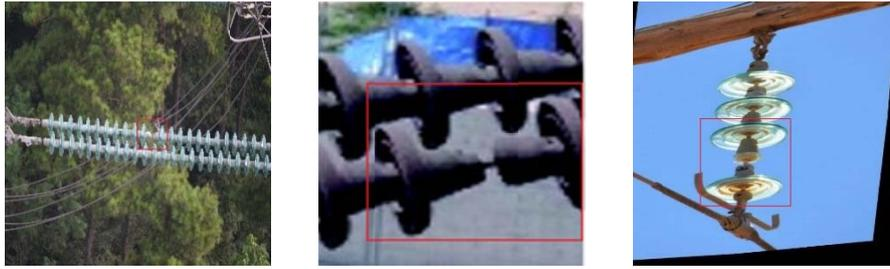
(b) Self-explosion defect insulators
