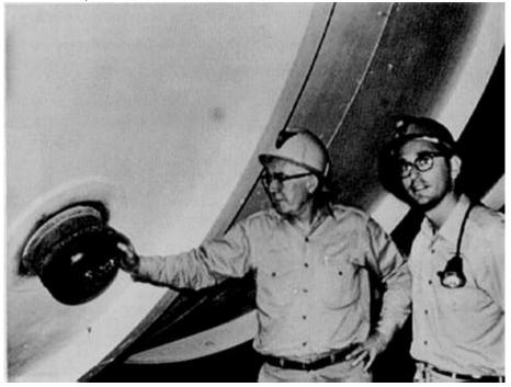
Ray Davis shows John Bahcall the tank containing 100,000 gallons of perchloroethylene. The picture was taken in the Homestake mine shortly before the experiment began operating.
