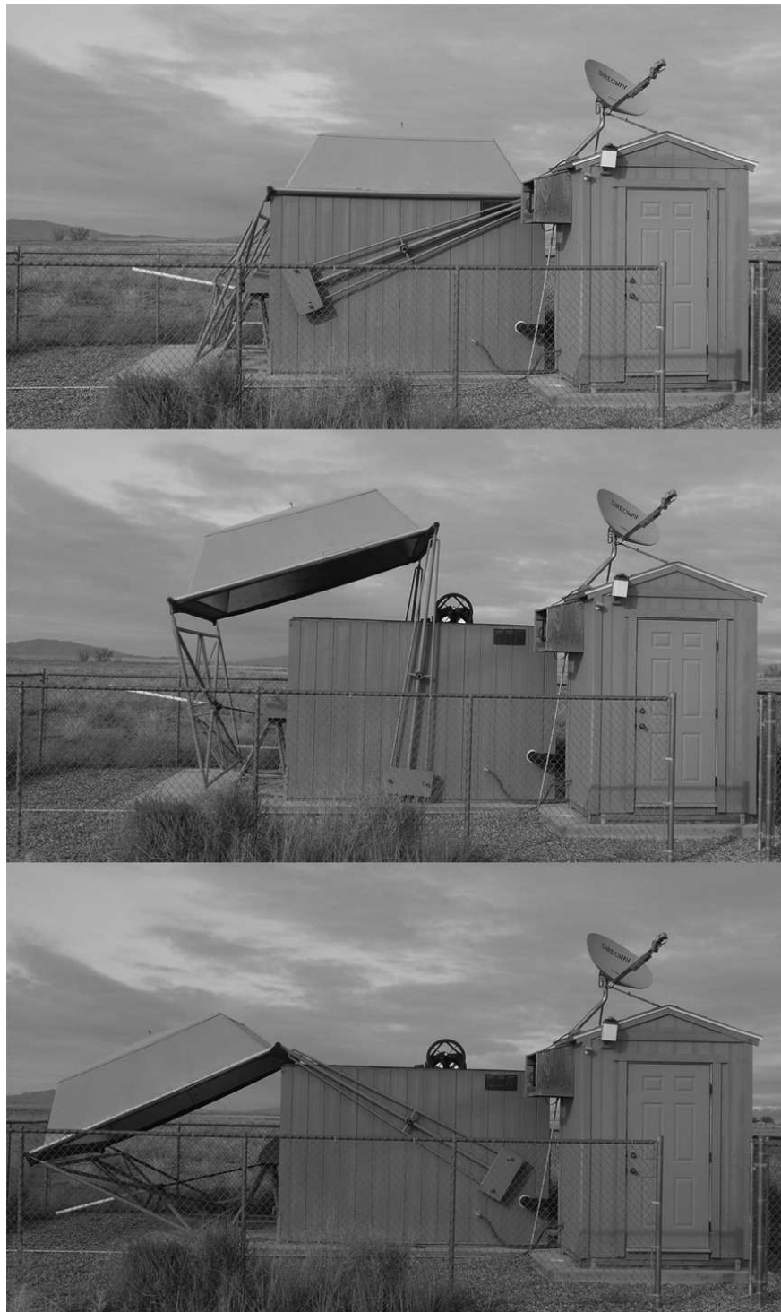
Fig. 2.— The ROVOR facility showing the roof closed (top), partially opened (middle), and fully open (bottom). The roof lifts up and over the telescope then lowers to allow the telescope an unobstructed view to within approximately 10 degrees of the western horizon. The electronics shed (called the “outhouse”) containing the communication and control hardware is on the right. The roof pull-off mechanism is on the left side.
