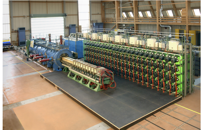
Fig. 1. PEGASUS railgun installation.
