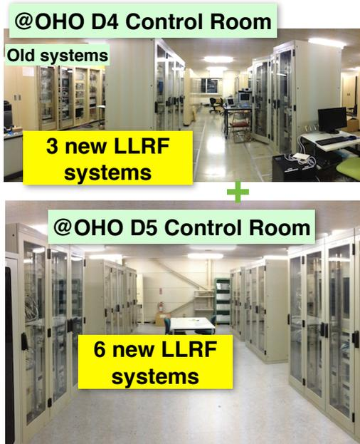
Figure 6: Installation appearance of the new LLRF control systems in the RF control rooms at D4 (upper) and D5 (lower) section.
