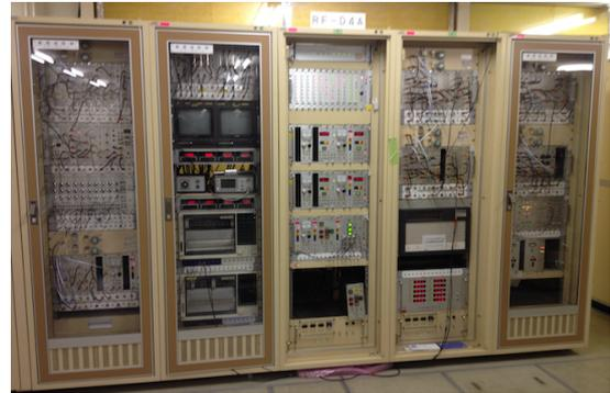
Figure 7: Old LLRF control system, which was used in KEKB operation, continues in use for SuperKEKB.
