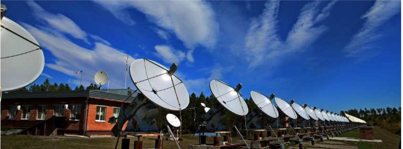
Figure 2: View of the 48-antenna SRH first stage (the east arm). White remote larger dishes on the right (east) belong to the old SSRT antenna system. Separate dishes on the ground behind the SRH antennas belong to the total-flux spectropolarimeters (Zhdanov and Zandanov, 2015). The receiver and control systems are located in the working building visible behind the SRH antennas on the left.
