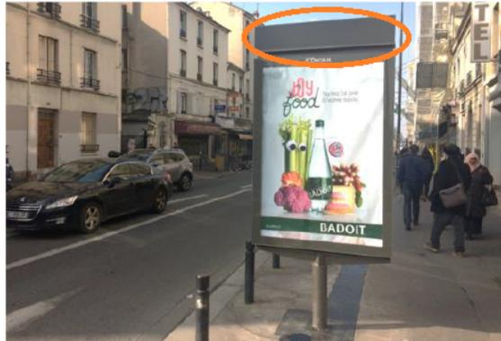
Figure 1: SC deployed on top of an advertisement panel
