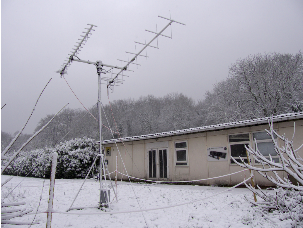
Figure 4. A view of the UHF/VHF antenna of the PicSat Operation Center, in Meudon, France.
