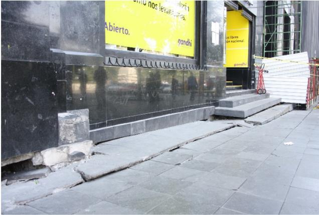
FIG. 16. Evidence of soil-structure interaction in Mexico City (Photo courtesy of S. Brûlé and A.F.P.S. [81]).
