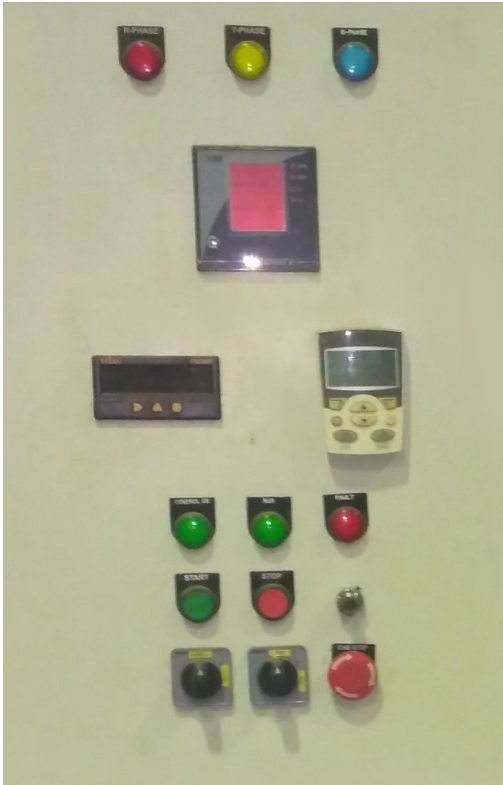
Figure 3: The electrical control unit for controlling the RPM of the pump.
