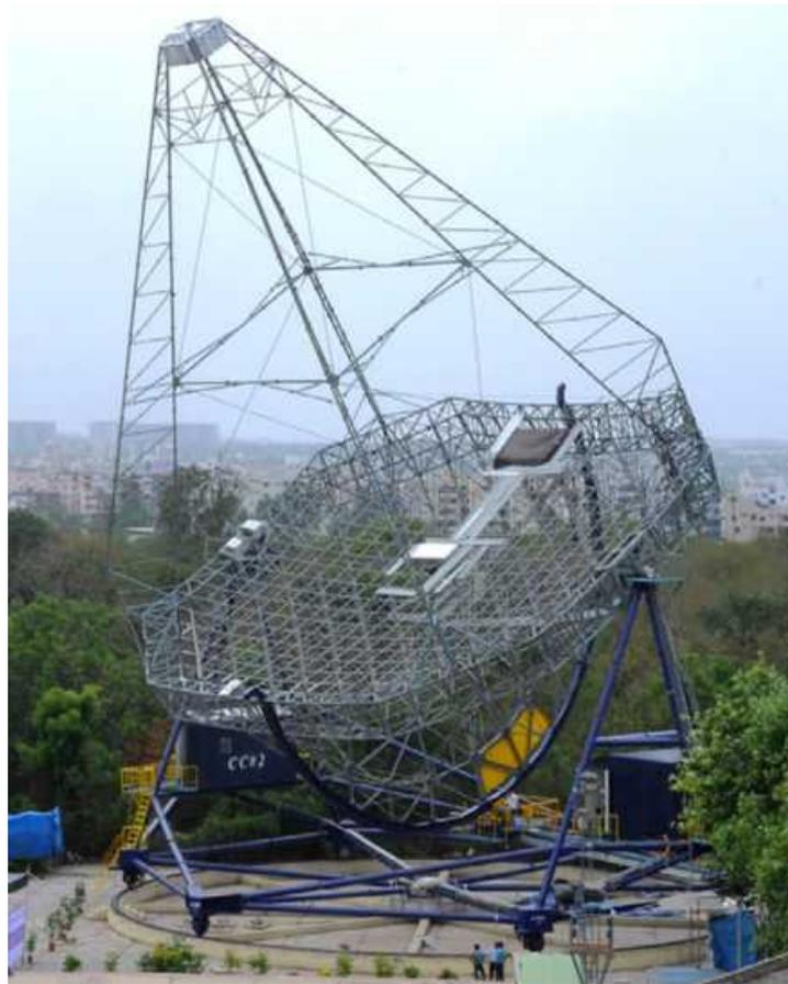
Figure 19.17: Figure taken from [Borwankar et al., 2016]. The MACE telescope has 21.3 m effective aperture-diameter. Here it is at its production site in Hyderabad before it is moved to Hanle at 4,270 m a.s.l..
