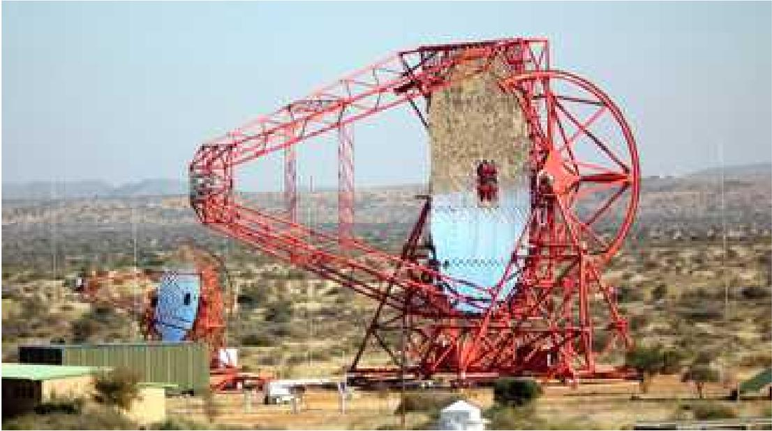
Figure 19.16: Figure taken from [H.E.S.S. collaboration, 2018]. The large H.E.S.S. II Cherenkov-telescope with 28 m effective aperture-diameter.
