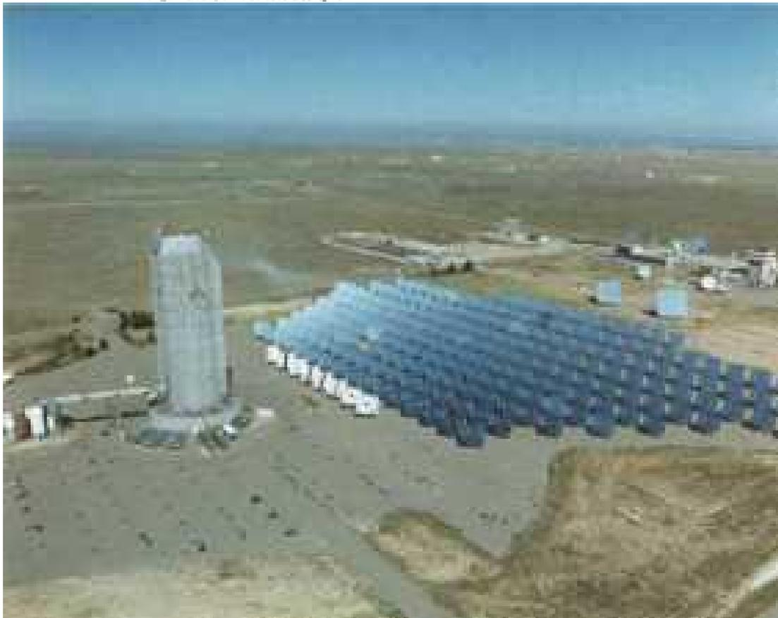
Figure 19.5: Figures taken from [Covault et al., 2001, Chantell et al., 1998]. The STACEE solar-concentrator for dense areal-sampling. The upper drawing shows the canting of the mirror-facets. Cherenkov-light reaches different mirrors (heliostats) on ground but was produced in the same point.
