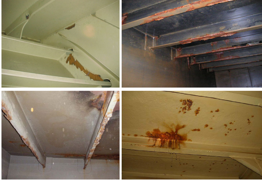
Figure 2: Targets to be detected in the visual inspection application case. The different images show examples of CBC on ship surfaces.
