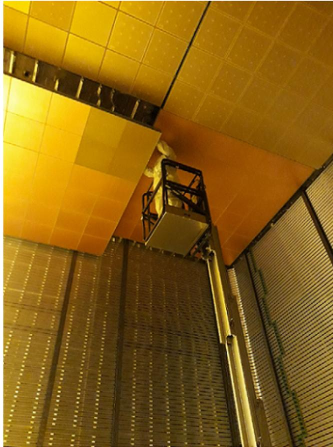
**Figure 47.** Installation of the last of the four CRP units into the ProtoDUNE-DP TPC. Connection of the readouts to the corresponding signal feedthroughs was performed in-situ as each CRP unit was moved into its final position. Taken from [82].
