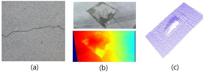
Fig. 3. Example snapshots of data collected from various sensors, including RGB cameras, stereo cameras, and Time of Flight (ToF) based depth sensors: (a) An image from the CrackForest dataset [46] taken by an iPhone 5's mobile camera. (b) An image of a road surface and the corresponding disparity map obtained by Fan *et al.* [53]. (c) Visualisation results of point clouds collected by Zhu *et al.* [54].
