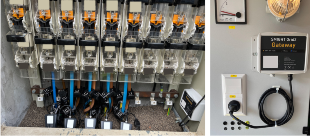
Figure 2: Example for sensors and gateway used in the MV/LV substations to measure the LV feeders. (image: Netze BW GmbH)
