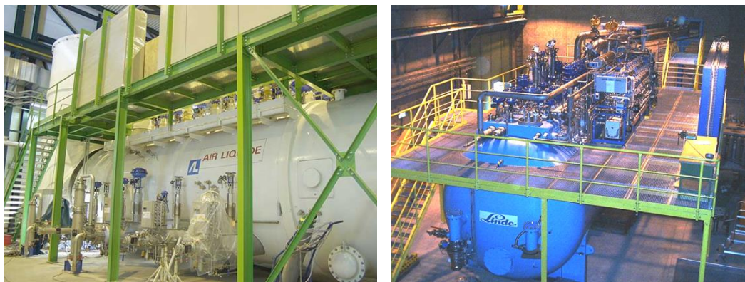
Figure 7. 18 kW at 4.5 K refrigerators (AIR LIQUIDE and LINDE) at LEP/LHC in the 1990s
