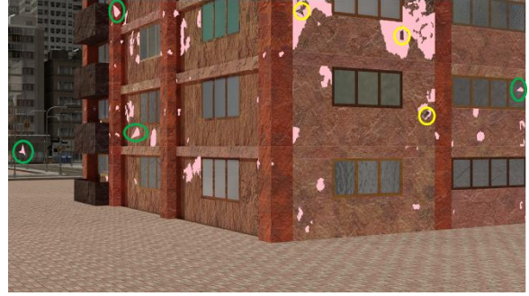
(b) modified spalling segmentations
