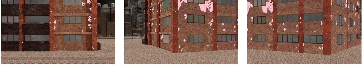
Figure 7. Examples of spalling-segmented images
