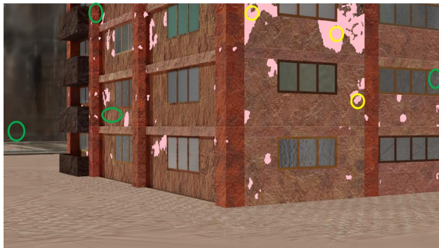
Figure 13. A spalling-segmented image rendered from the 3D GS model presented in Figure 12
