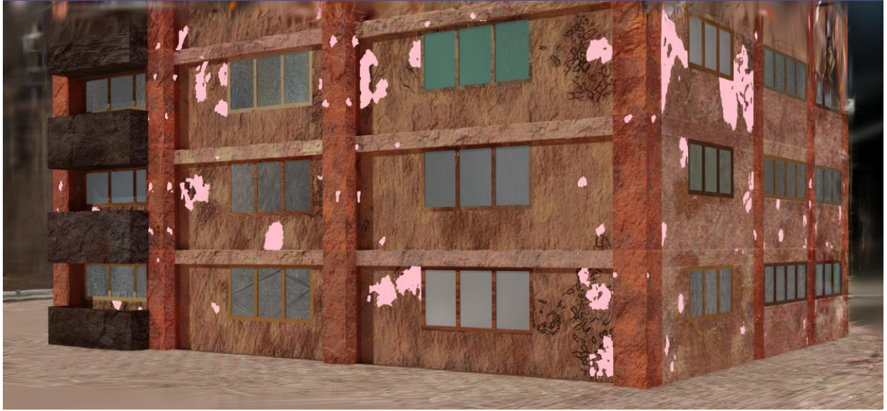
Figure 8. GS-enabled 3D damage visualization results using 60 spalling-segmented images
