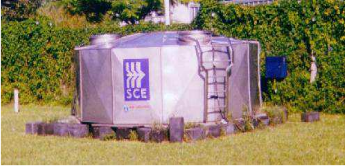
Figure 3: Detector B. The cabinet installed on the wall at the right side contains the local electronics and the high voltage power supply.
